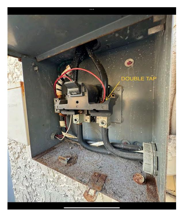
No main breaker inside the MSP to protect the loads of the home (the main breaker is larger than the other breakers in the panel). This is required by code:
